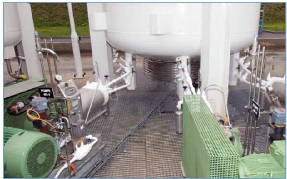
RVT with triple thermosiphon option and separate liquid offtake line
