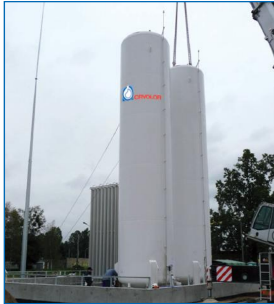
All tanks, from C3 to C77 are designed for one-crane erection to cut installation and handling costs.
